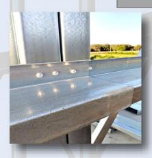
On site COLD FORMED main frame is typically both bolted and screwed together using pre-drilled plates. COLD FORMED buildings can require some cutting/coping and drilling of braces on site.
