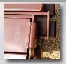
Structural steel has a painted finish typically in the red although can come in many colors. The paint is intended only to protect the steel during construction and transport and is easily damaged.
