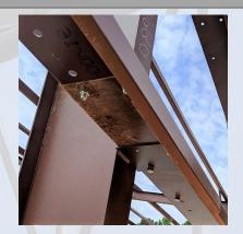
On site a Structural Steel main frame is typically bolted together with plates already welded in place in the factory. Structural Steel buildings can require some welding and drilling on site.
